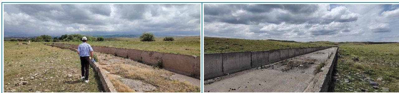
Figure 2-5. Existing G-20 type concrete channel
