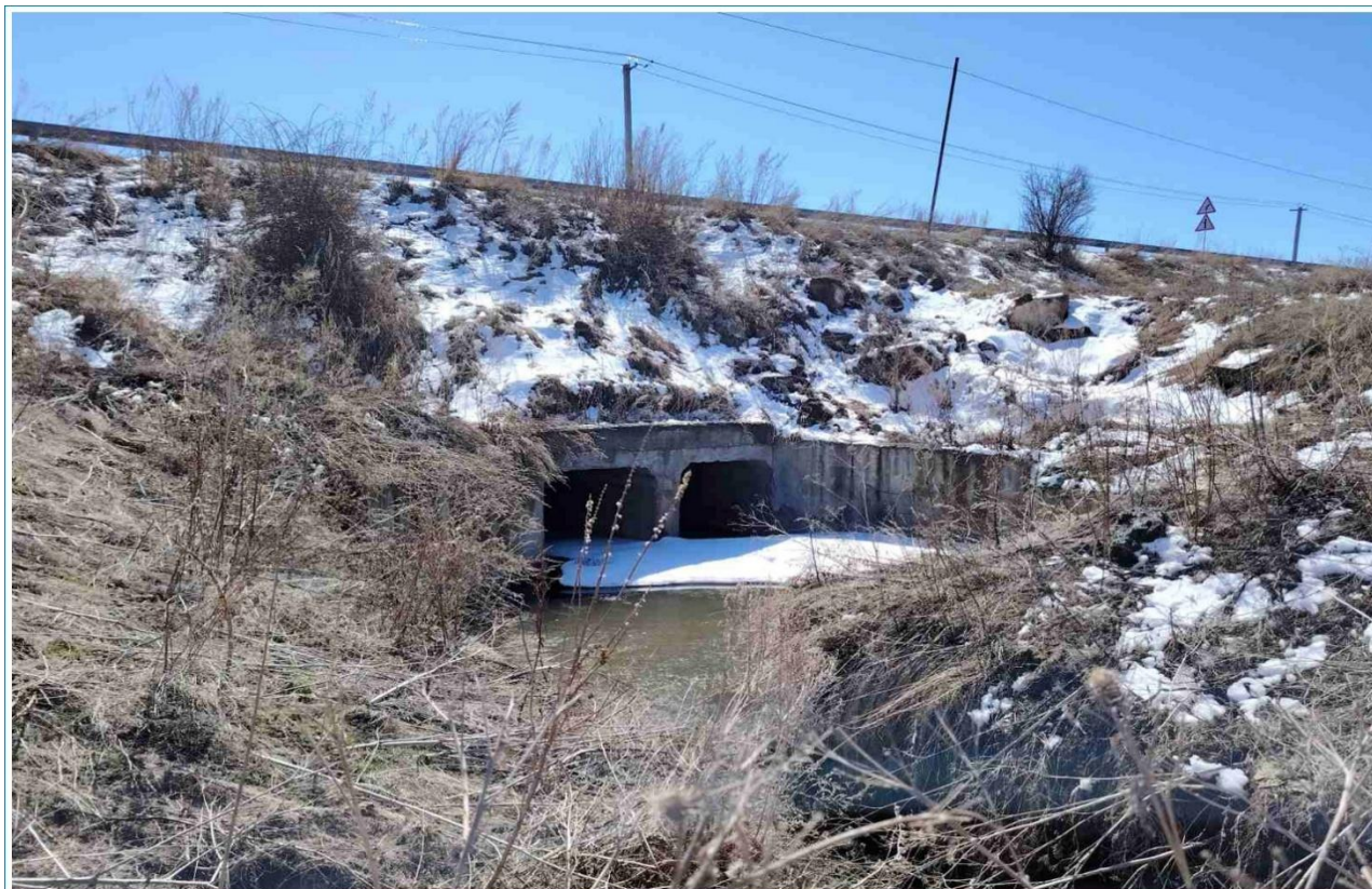
Figure 2-6. The existing twin-barrel tunnel under the Maralik-Artik highway
